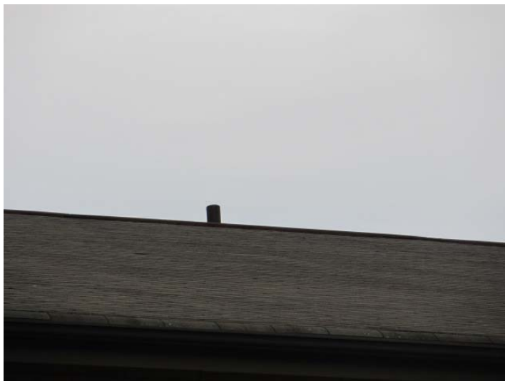
Original roof shingles are serviceable but have surpassed their expected useful service lives
