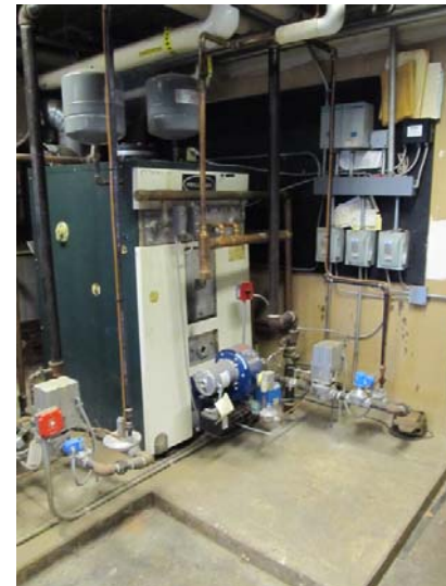
Domestic hot water produced by a single natural gas-fired boiler located in mechanical room at lower level of building
