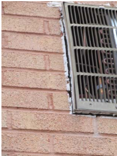
Caulking at perimeter of air conditioner sleeves also in need of replacement in near-term
