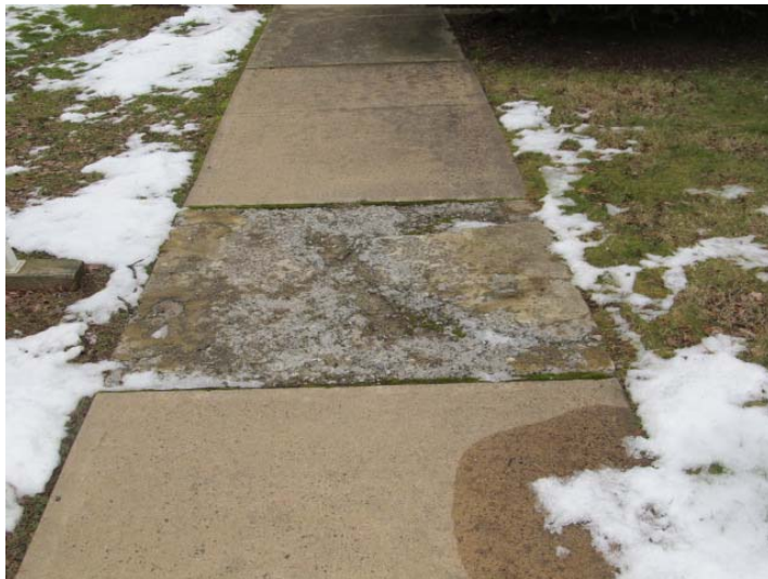
Sectional repair/replacement of walkways needed in near-term
