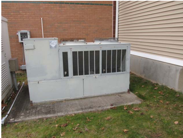
Exterior, air-cooled, chiller used to provide cooling for interior common areas
