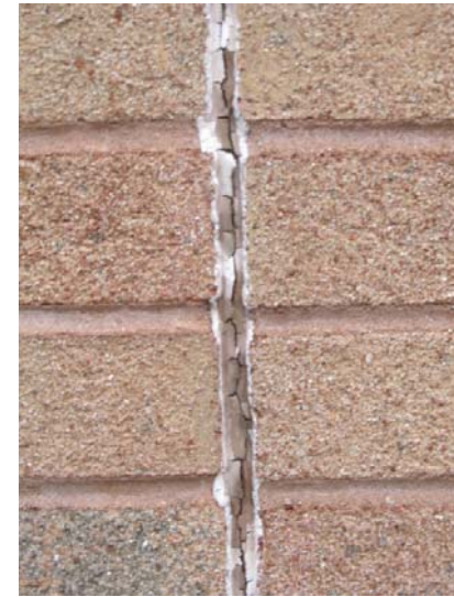
Caulking in control joints exhibits age-related loss of cohesion and pliability
