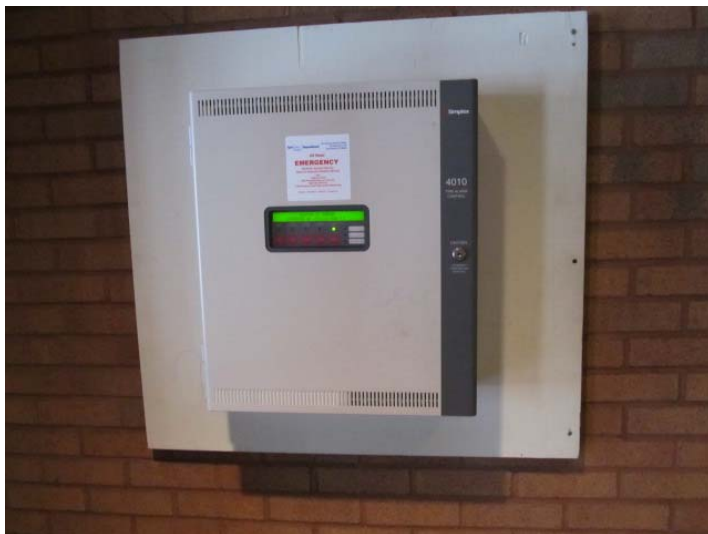
Fully addressable central fire alarm control panel – Equipment updated in recent years
