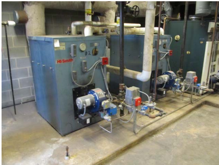
Natural gas-fired hydronic boilers for heating of interior common areas and dwelling units
