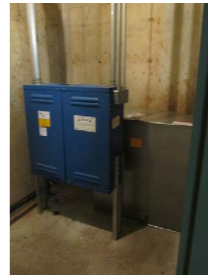
Elevator controller/dispatcher and hydro-mechanical equipment
